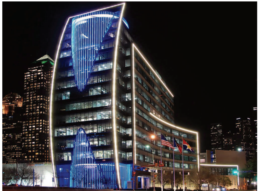
The façade of the Hunt Building in Dallas.
