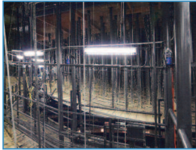
Figure 6: Guide tubes between grid and plaster ceiling.
