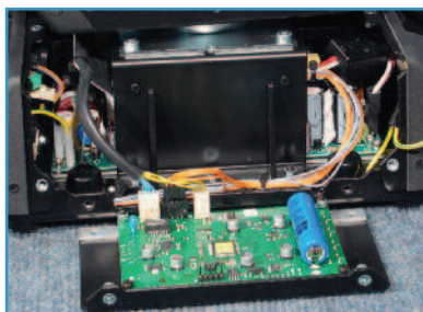
Figure 19: Control and power supplies
